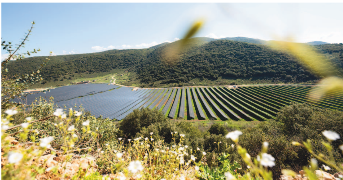
50 MW Margariti solar farm, Greece.
