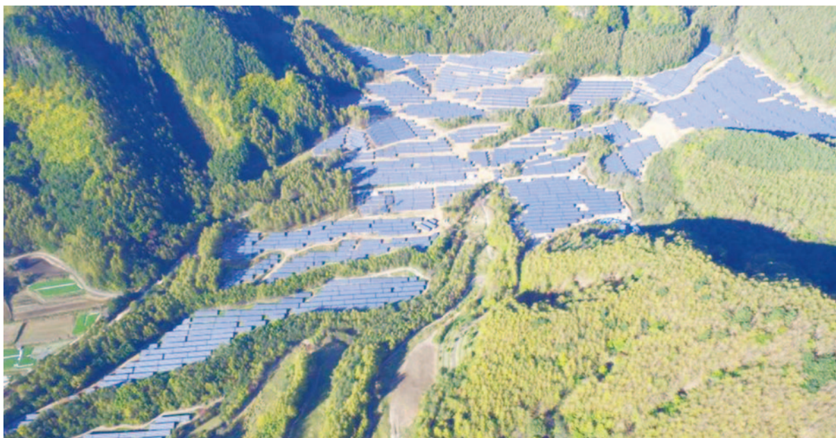
Kawakami-2 Mega-solar project, 31 MW, installed at an altitude of 1,600 meters, Nagano, Japan.
