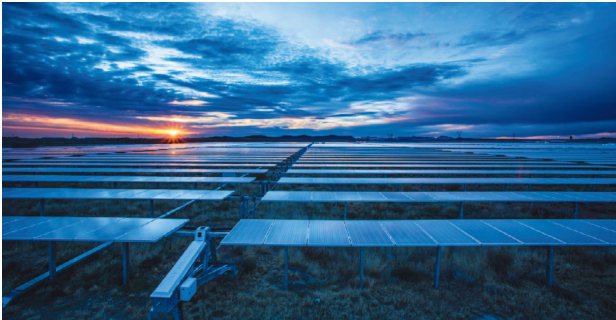
40 MW Linde solar farm, Northern Cape Province, South Africa.
